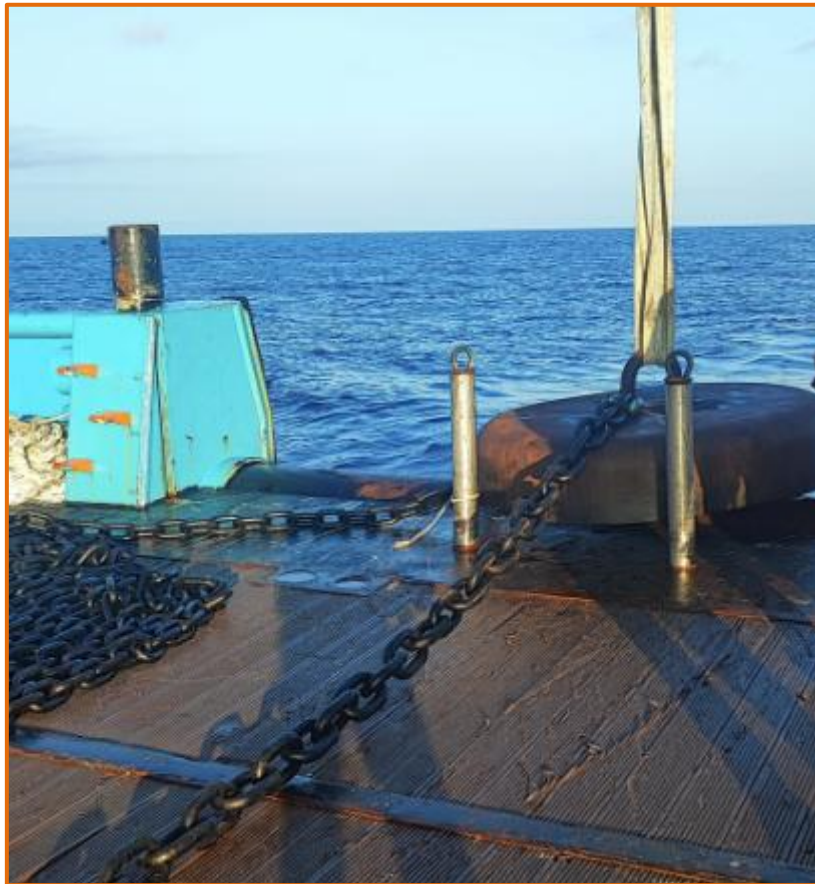
Figure 13: Clump weight being lifted using the vessel crane.
